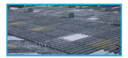
The use of Asbestos Cement (AC) was banned in new buildings in 1990 due to growing concerns about the health hazards posed by asbestos fibre release, especially during construction and maintenance.
